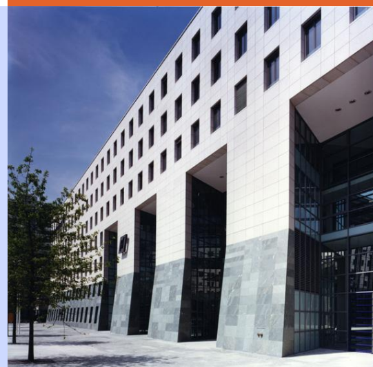
IKB headquarters in Duesseldorf
